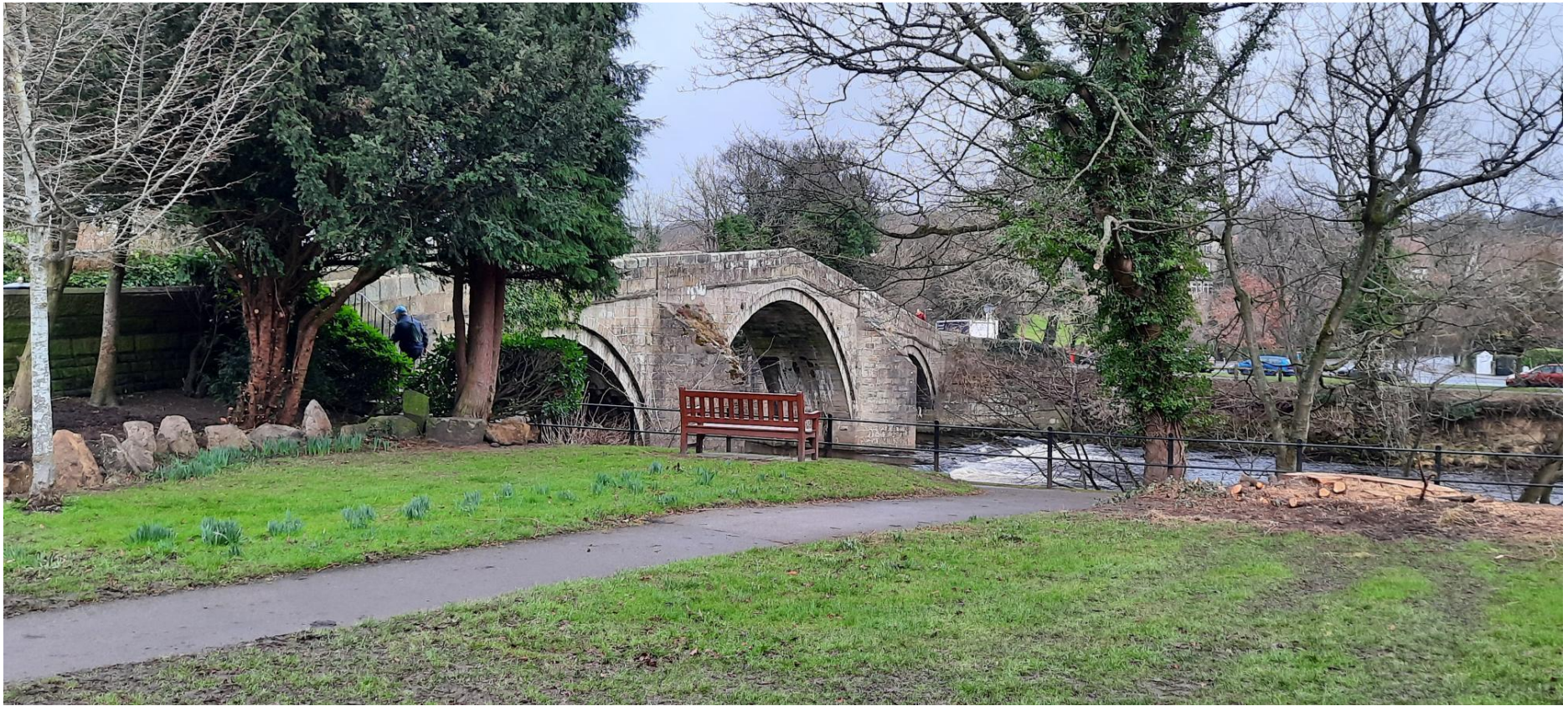
Ilkley Old Bridge, scheduled monument as seen from Bridge Lane, immediately to the north of the site
