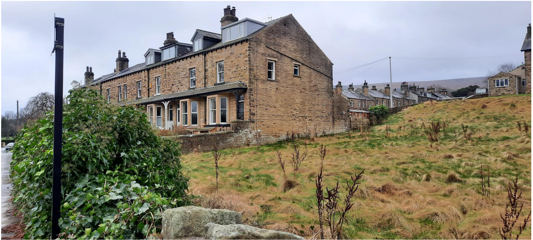
View from Bridge Lane eastwards to 41-53 Bridge Lane
